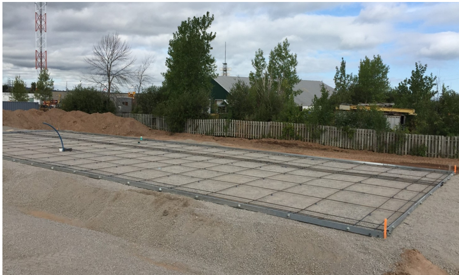
DESIGNED AS A SUSPENDED SLAB, INVERTED, USING 150 GRADE HIGH-YIELD POST TENSION BAR UNDER COLUMN AND IN A STRUCTURAL SLAB GRID CREATING A 2-WAY REINFORCED CONCRETE AS A STRUCTURAL FOUNDATION SUPPORTING SUPER-STRUCTURE LOADS, ON GROUND.
