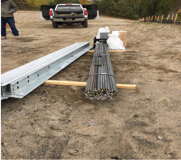
PRE-FABRICATED DIMENSIONALLY STABLE EXTERIOR FORM CHANNELS WITH PRE-DRILLED PERIMETER BEAM BAR AND SLAB GRID BAR SLOTS
